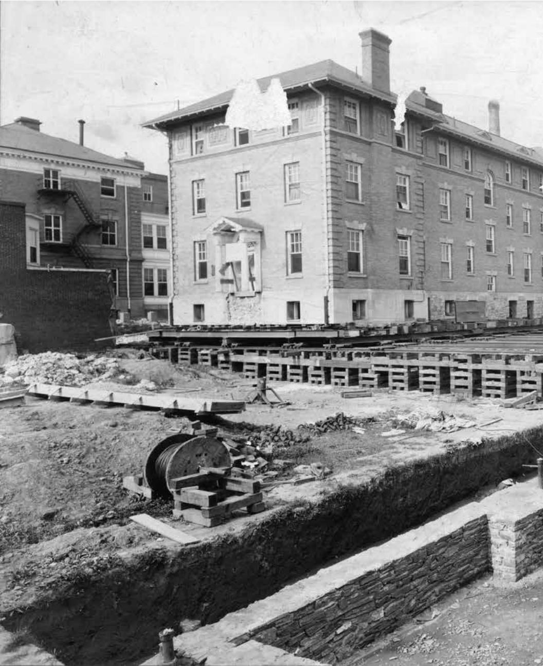
Moving FonDersmith Nurses' Home to make room for new maternity wing along North Lime Street, c. 1927. LHO 2011108
